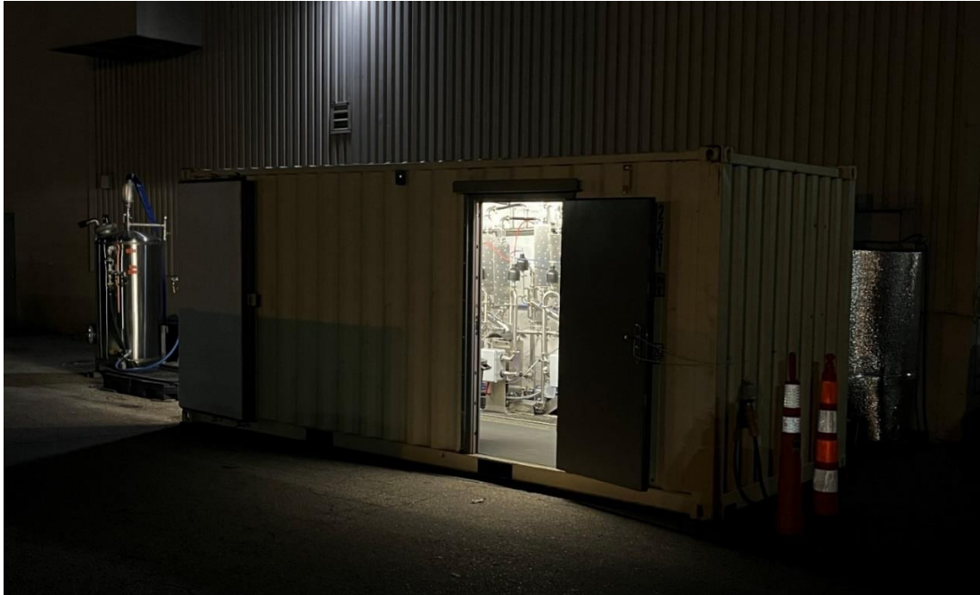
Night-time AMEOX® processing of PFAS in Granular Activated Carbon (GAC) within in standard size water treatment cell (left) (WRS, Wyoming, MI – October 2022)
