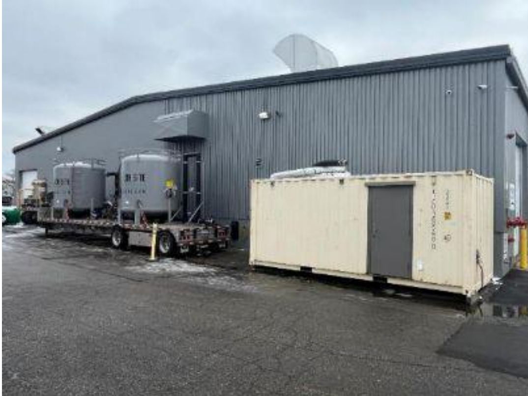
2 x 10,000# Trailered GAC (right) Absorbers (left) AMEOX Dual Unit in 20' Shipping Container
